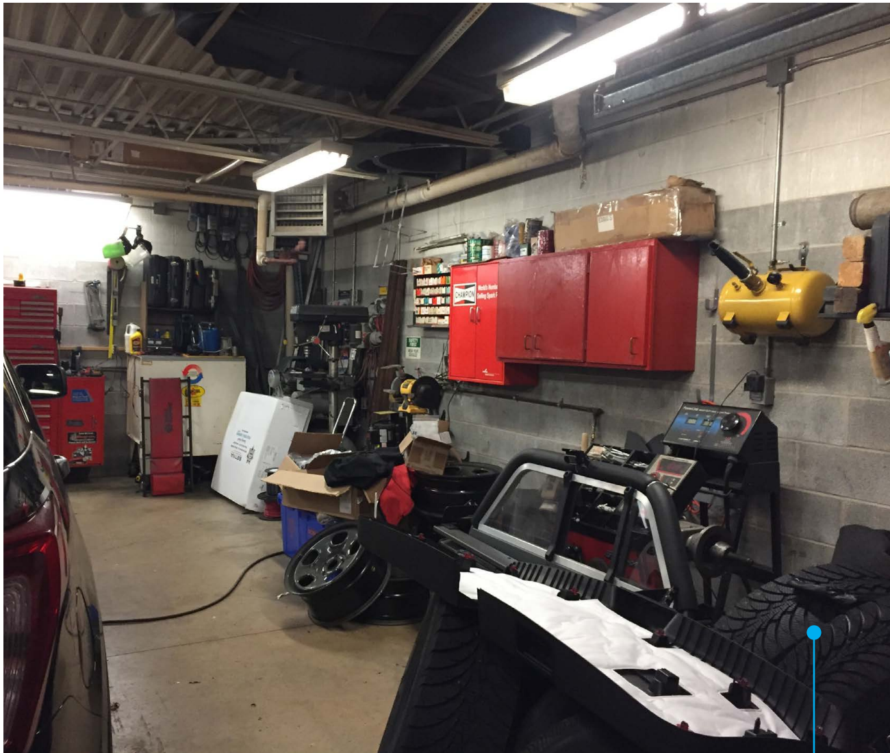
MAINTENANCE GARAGE: NOT ENOUGH SPACE IN MAINTENANCE GARAGE AREA FOR GENERAL STORAGE; THERE IS ALSO A LACK OF VENTILATION IN THIS SPACE WHICH IS NOT AN IDEAL ENVIRONMENT FOR EMPLOYEES.
